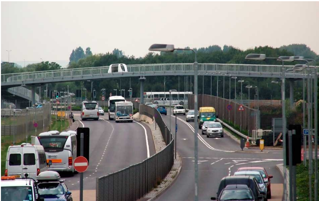
Figure 1.2: Photograph of an elevated two-lane PRT guideway section at London Heathrow Airport. Nominal guideway elevation over a main road is 5.7m (18' 8"). An ULTra vehicle is moving on the guideway, just left of the central column. Photo courtesy of ULTra PRT Ltd.
